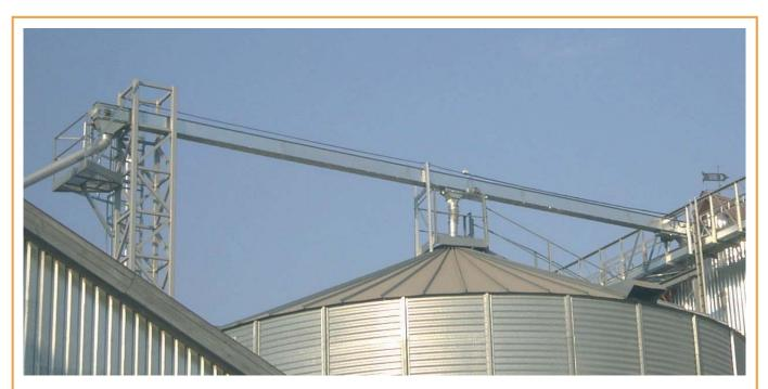
The **PETKUS Troughed chain conveyors** are well suitable for the conveyance of bulk material in the agriculture and industry, like cereals, oil seeds, pulses, as well as for the transport of products in powder form.
